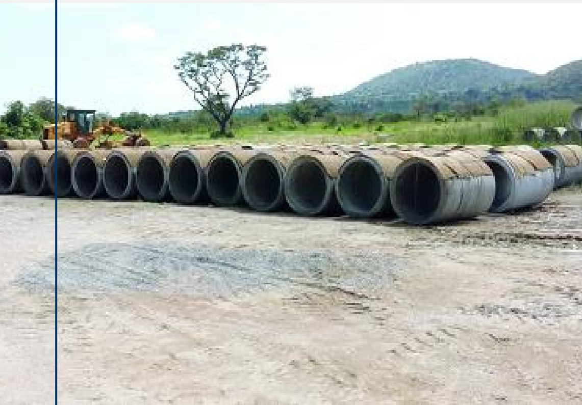
Production of pre cast yard precast pipe culverts at the
