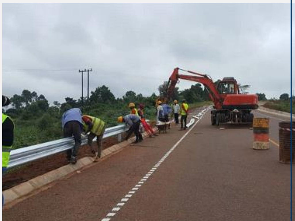
Installation of guardrails on Kanoni- Sembabule-Villa Maria Road
