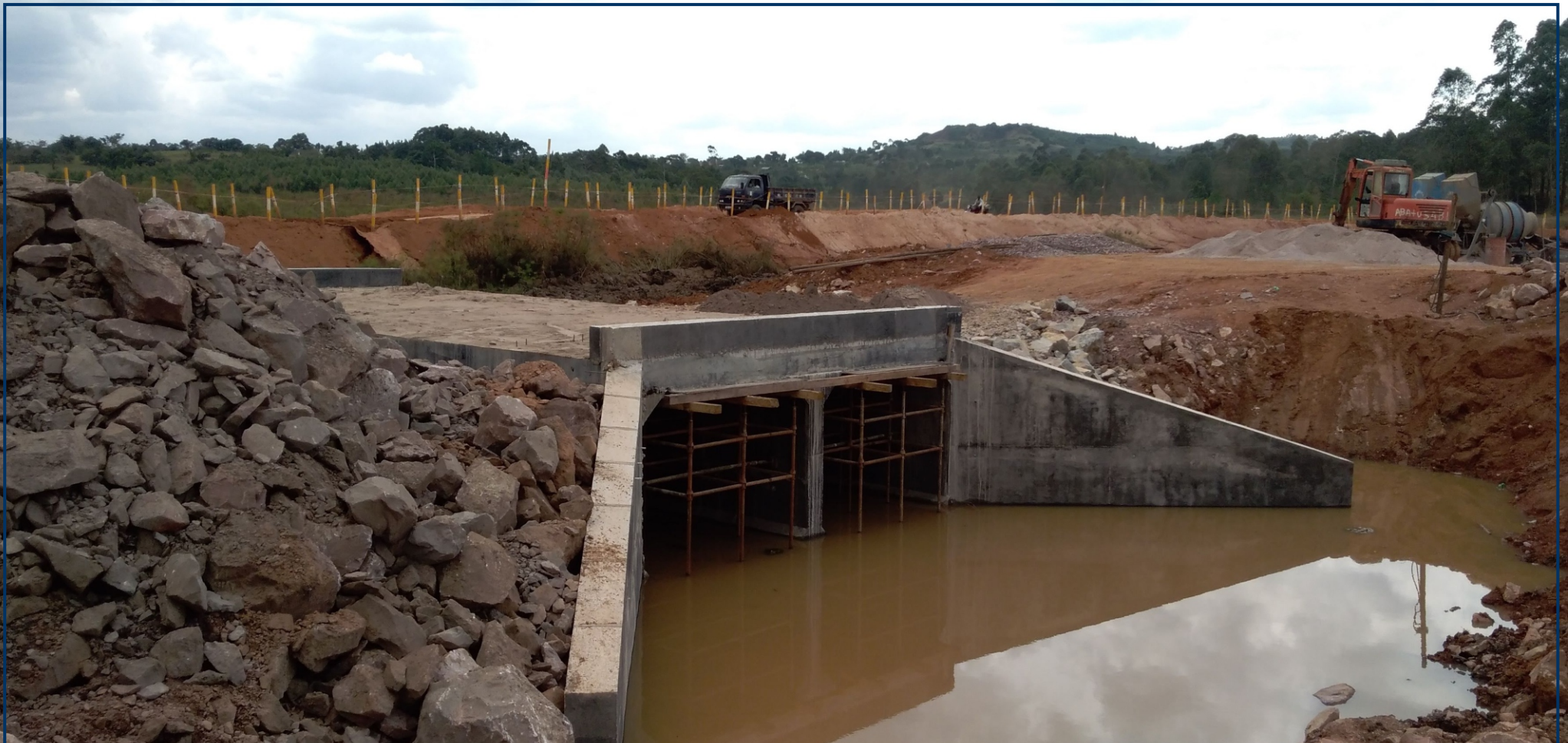
Construction of a box culverts along Kanoni- Sembabule-Villa Maria road project (110km)
